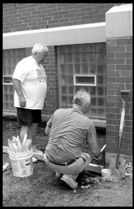
Joe Calamante and Patrick Racut prepared the forms for the concrete walks in the rectory gardens.
