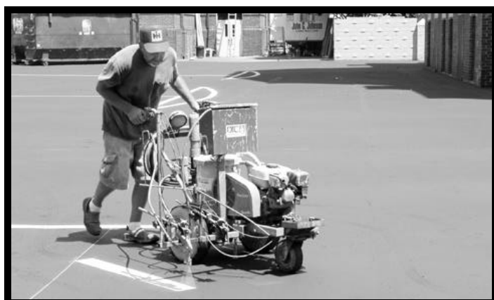
Parking lot resurfacing was completed on Monday of last week.
