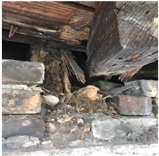
Approximately 70% of rafter tails are deteriorated on North side
