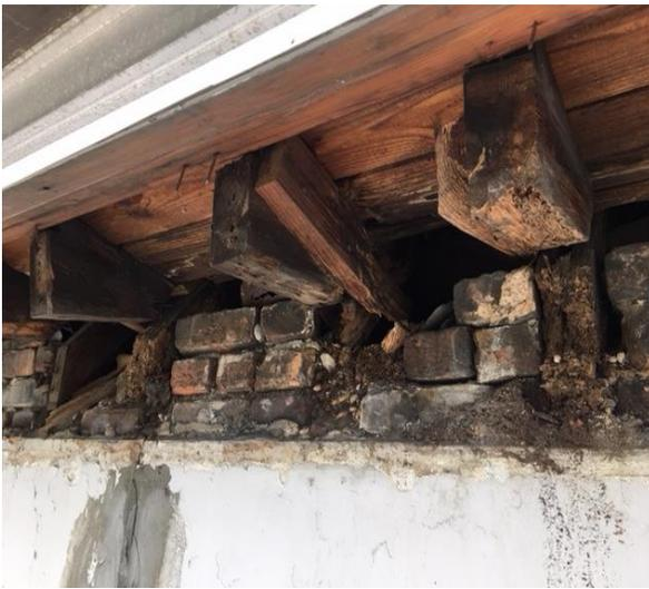
“Typical” deteriorated conditions behind upper roof cornice
