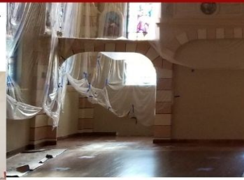
Above: The area before the construction of the new confessional
