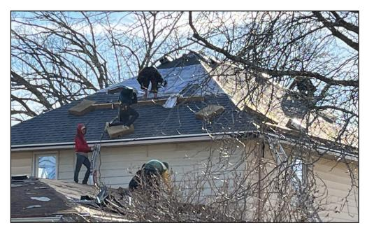
**DURING:** Workmen from Butler-based "Rescue My Roof" removed old shingles, installed new baseboards, and re-shingled the roof.
