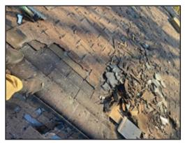
**BEFORE:** Loose shingles, gaping holes, crumbling tiles were everywhere — it's no wonder that, at one point, bats managed to find their way into the attic. When heavy winds combined with rain, water leaked into Father Sergio's bedroom. Roof work is costly and the repair work was postponed more than once. This fall's storms were the last straw.
