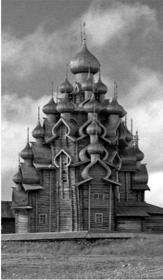
**Transfiguration Church** is on Lake Onega in Republic of Karelia, Russia. The 1714 structure itself has 22 domes and constructed with thousands of pine logs and no nails. Legend has it that the builder used one axe for the entire building, which he threw into the lake with the words “there will never be
