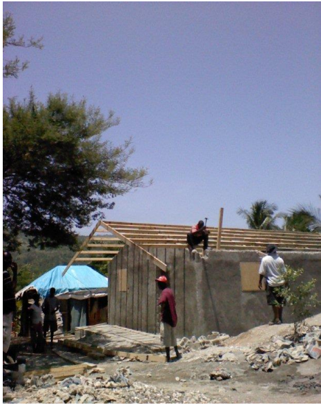
The roof goes up 2013
