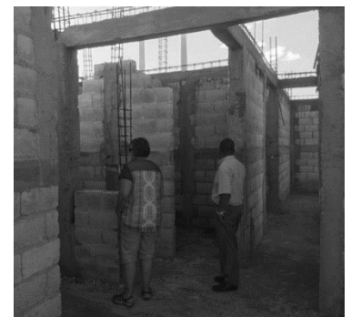
Progress on the new St. Anthony House
