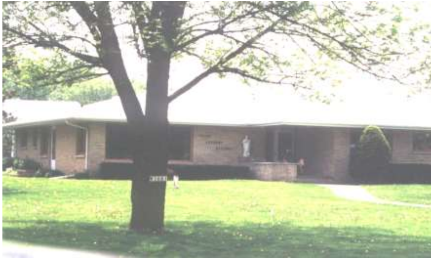
St. Andrew new rectory completed in 1965
