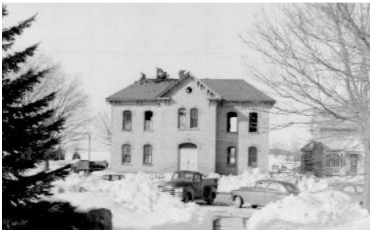
St. Andrew ` school being demolished by men of the Parish 1959 .
